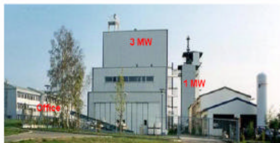
Gasifier Reactor with cooling wall 2-3 MW max. 30 bar Pulverized fuel dosing and feeding system up to 10 t/h Inert gas plant 1000 m 3 /h 80 bar Oxygen plant max. 300 m 3 /h 80 bar Slurry feeding 300 kg/h Sewage sludge drier 50 kg/h Pyrolysis unit 50 kg/h SulFerox desulfurization unit Waste water treatment CO 2 hydrolysis HCN hydrolysis
